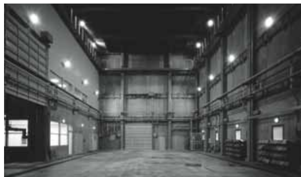
15m×30m×15m[H] (450m 2 6,750m 3 ) 放水能力：最大4,000L/min(0.98MPa)
